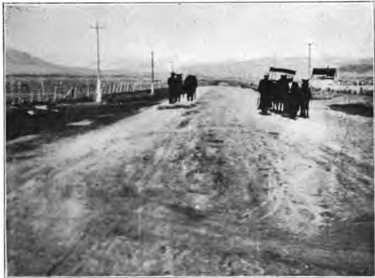
FIG. 10. SAME AS FIG. 9, AFTER WORK OF CONSTRUCTION WAS COMPLETED. SHOWS SPLIT LOG DRAG IN OPERATION
